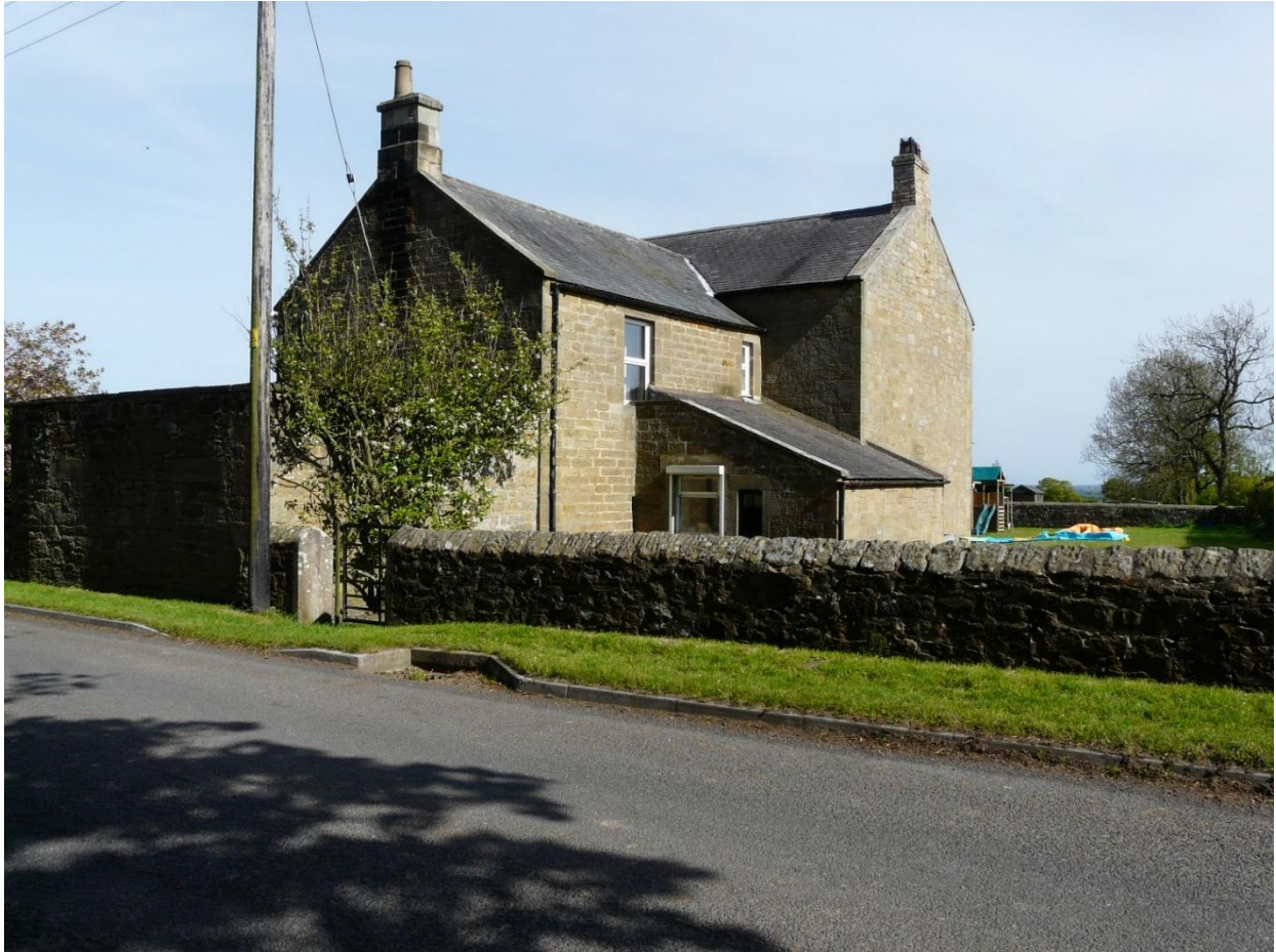
Plate 12: View of High Highlaws Farm from the road
