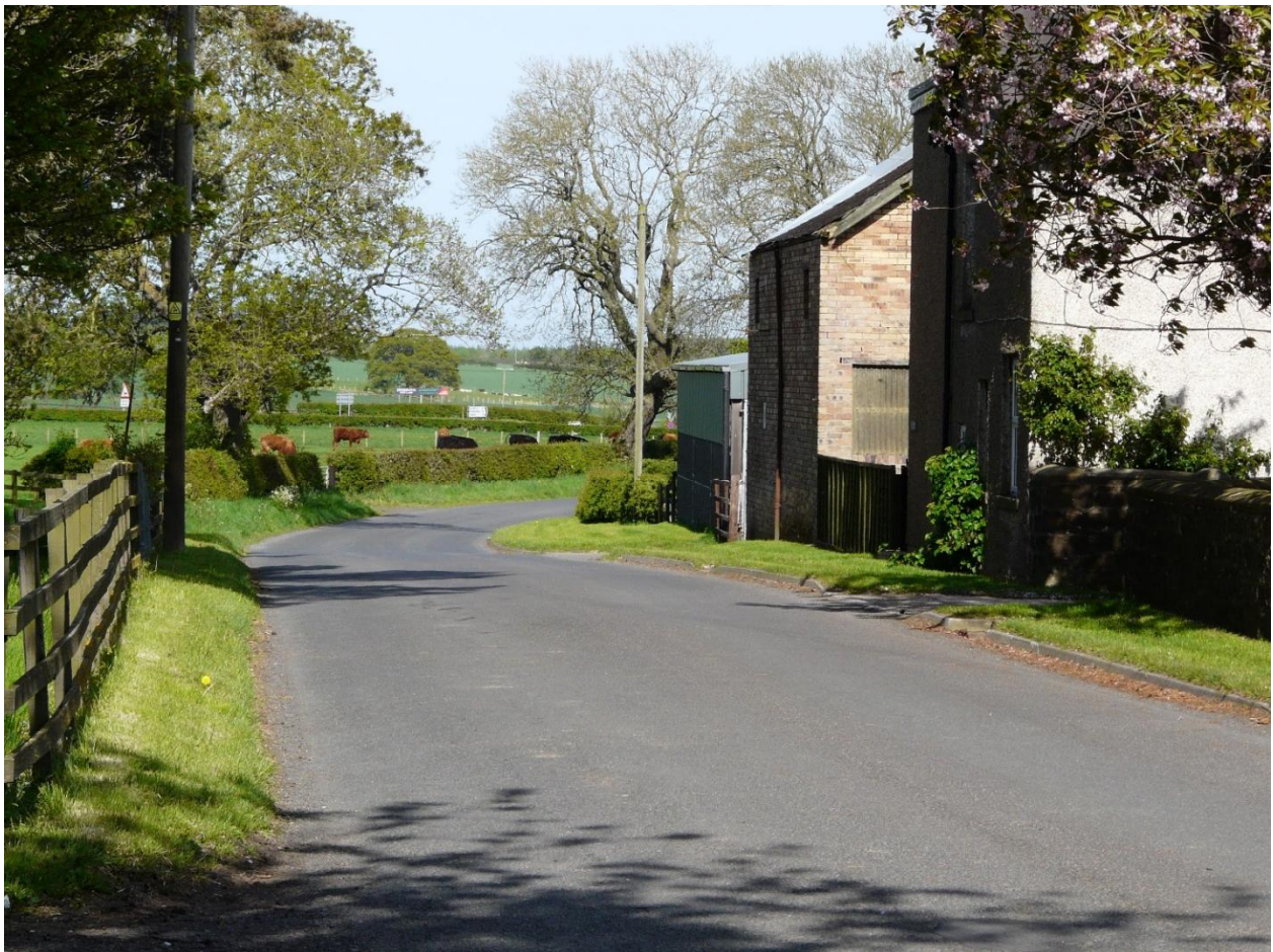
Plate 11: View from High Highlaws Road to the A1 and the area of proposed works for the junction
